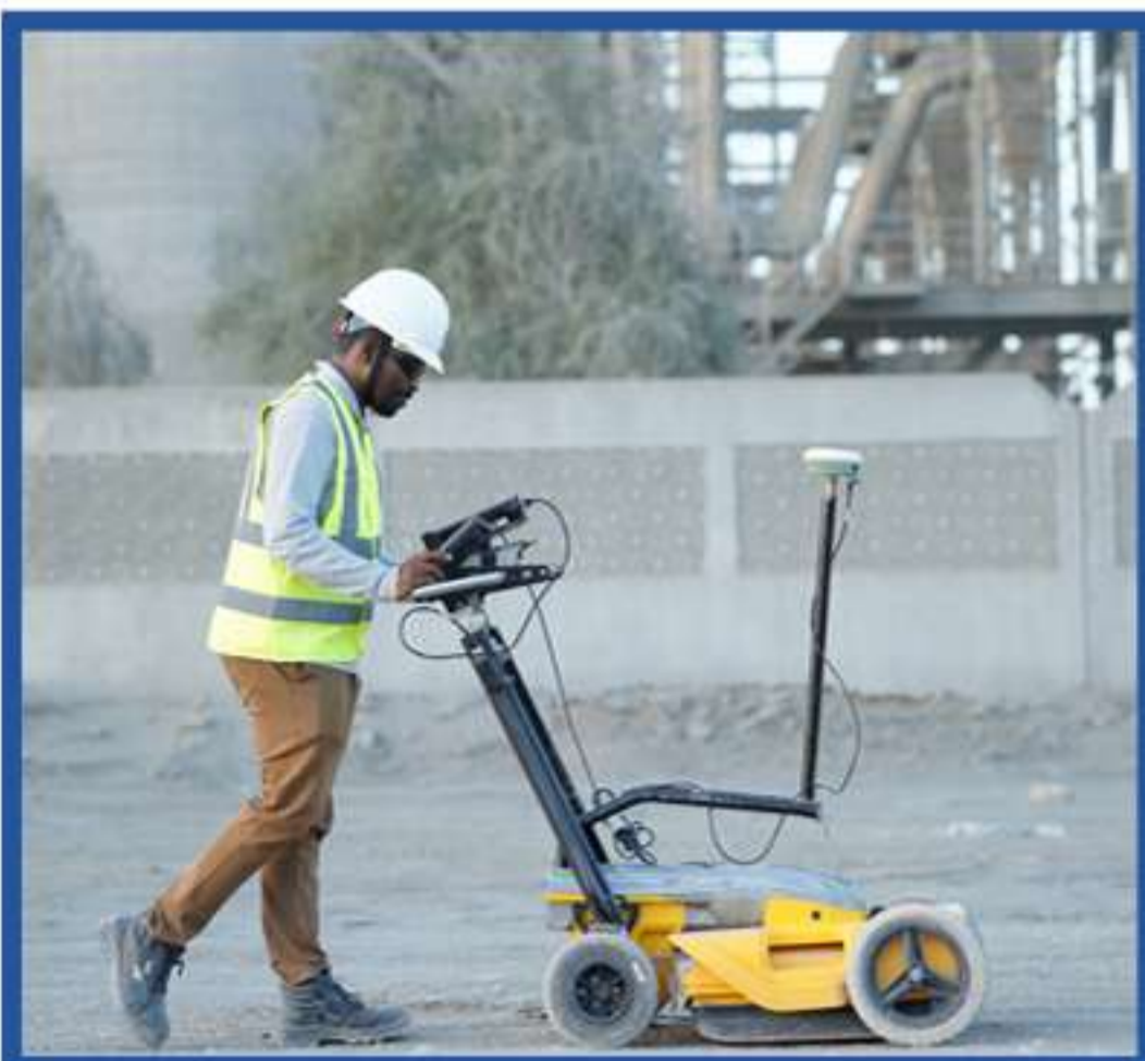
Under Ground Utility Scanning
